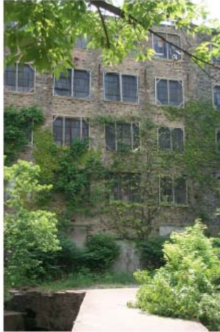
Historic Kent Mill Structure in the Proposed Upper Darby Area Greenway
