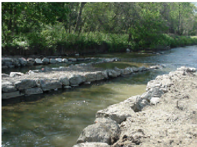
Giant stone weir in Darby Creek at Bartram Park provides habitat for fish.
